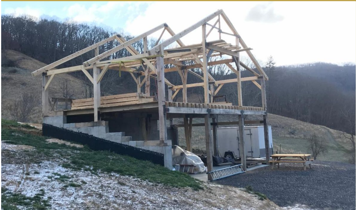
New workshop being constructed at Tonoloway Farm in Highland County.
